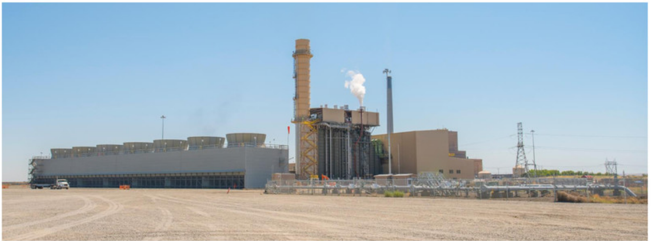
Carty Generating Station, a 440 MW natural gas baseload plant near Boardman, OR
